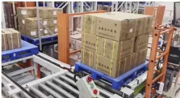
Automated Stereoscopic Warehousing System
