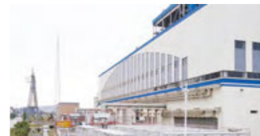
The first World Bank-financed battery energy storage project in the Guangdong-Hong Kong-Macao Greater Bay Area
