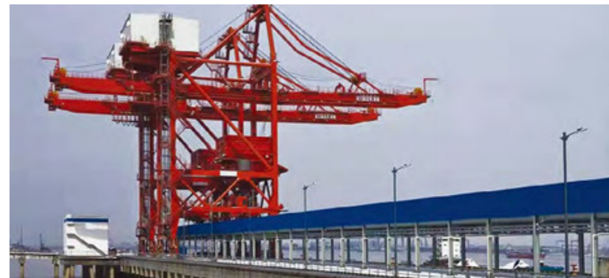
An energy supply project supported by Nanjing Branch
