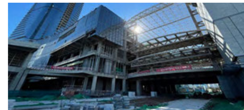
The Bank supports the construction of Beijing Municipal Administrative Center
