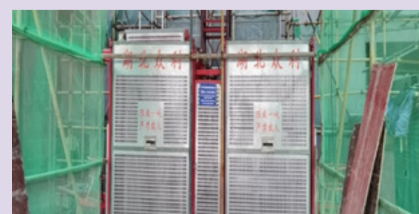
Hubei Linglong inspects the special equipment (elevators) on the construction site
