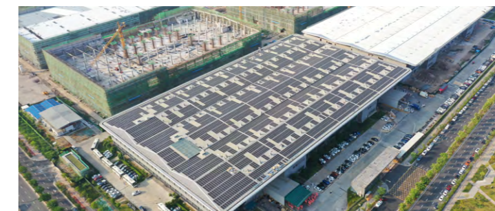
Midea MCA's Integrated Solar and Storage Demonstration Project
