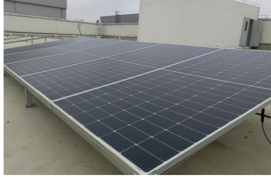
Site of "Lotus" module in Hefei factory
