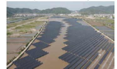
Tidal and light complementary photovoltaic power plant
