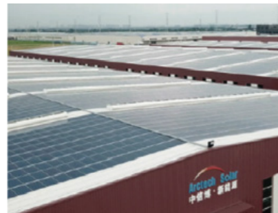
Exterior view of the BIPV roof of the plant
