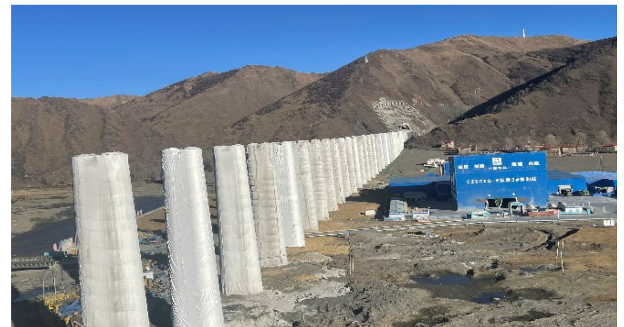
Sichuan-Tibet Railway construction site
