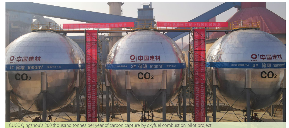
CUCC Qingzhou's 200 thousand tonnes per year of carbon capture by oxyfuel combustion pilot project
