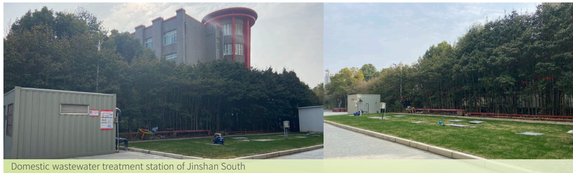
Domestic wastewater treatment station of Jinshan South
