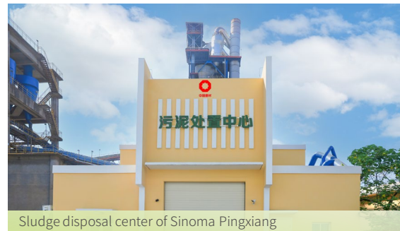
Sludge disposal center of Sinoma Pingxiang
