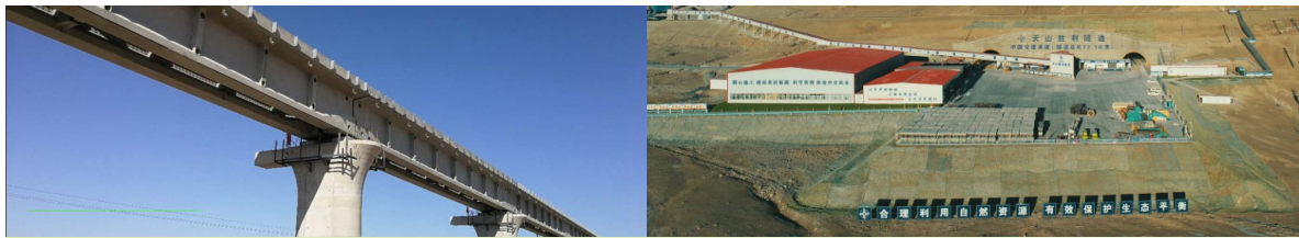
Construction site of Xinjiang Ge'ermu-Ku'erle Railway and Urumchi-Weili Expressway
