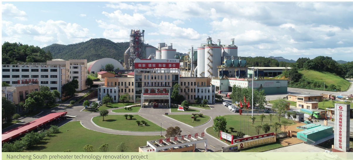
Nancheng South preheater technology renovation project
