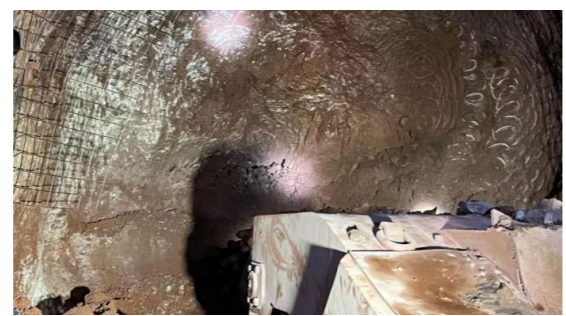
Boom-type roadheader promoting green and safe development of mining work
