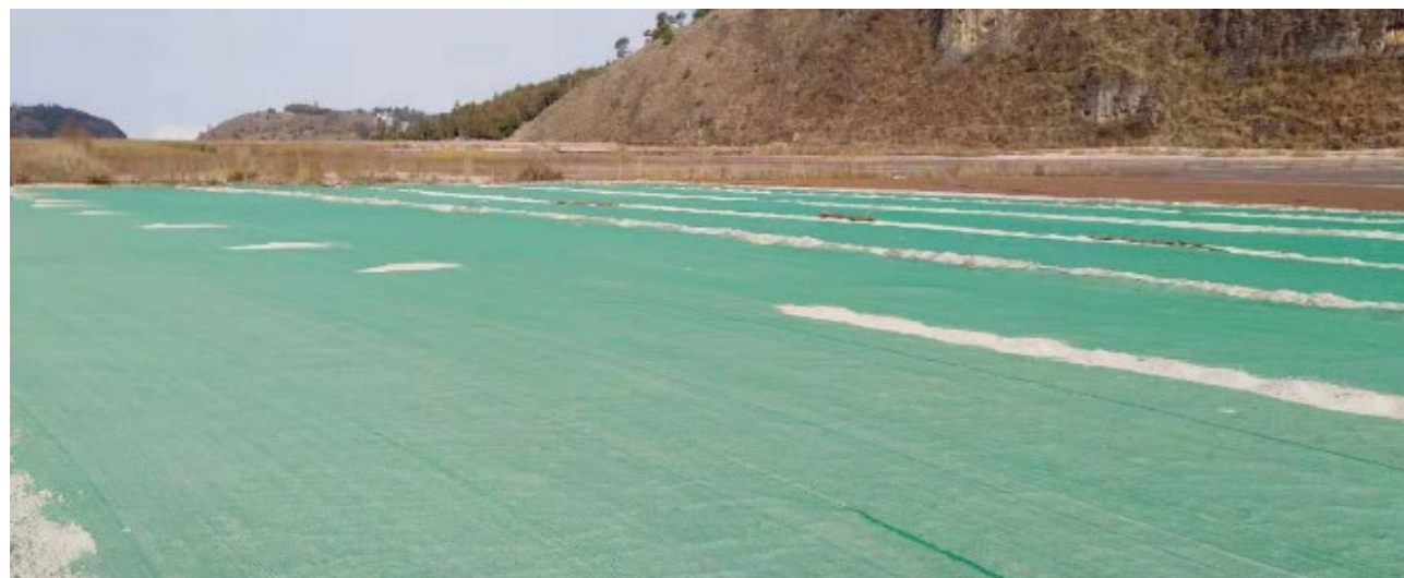
Dust-proof net laid on the dry beach of the tailings pond of the Laochang Branch
