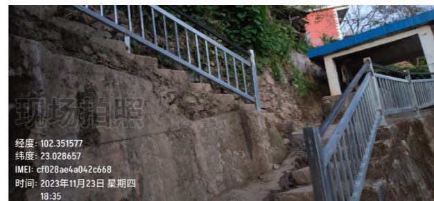
Repair of guardrail
