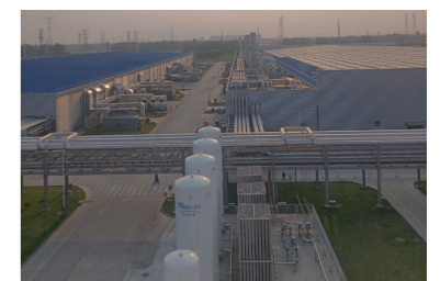
宿迁光电厂区环保配套设施
