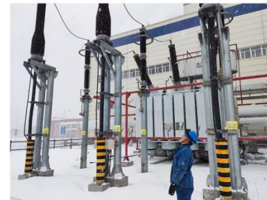
严寒天气检修
