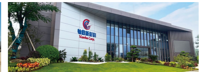
The Project of High-performance Paper-based New Materials in Sanjiangkou area, Laibin City, Guangxi
