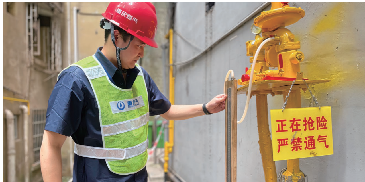
燃气抢险试压
