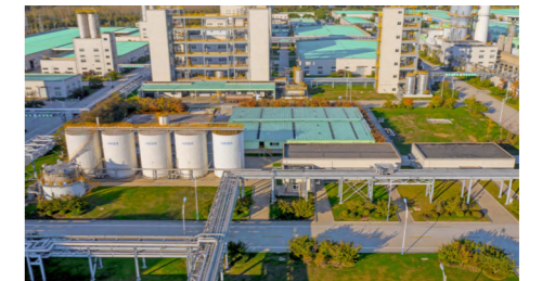
Biogas Power Generation Unit
