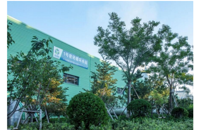
Closed Circulating Water Station No.1
