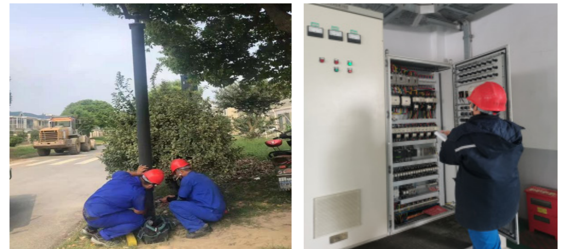
Line Maintenance in Kaisha Village
