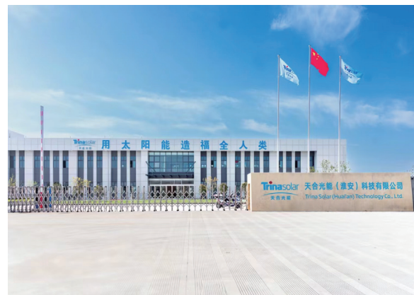
Trina Solar Huaian production base
