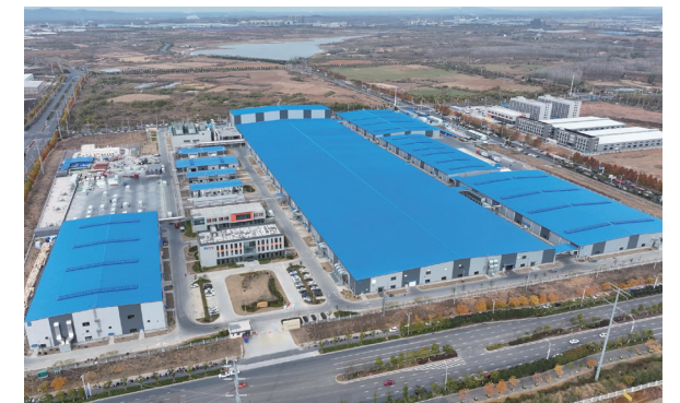
Aeroview of Chuzhou Storage Factory
