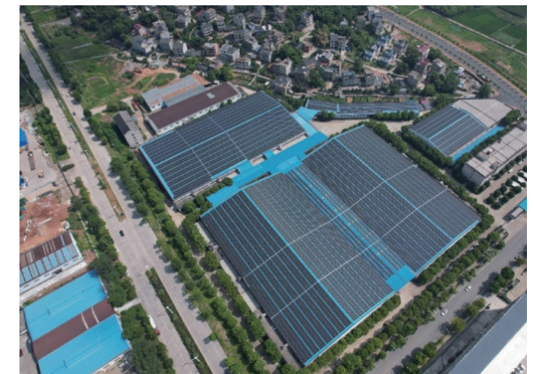
The rooftop PV project of Shangrao Delong Textile Co., Ltd.
