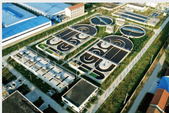
Industrial Cluster Sewage Treatment Plant in Luyi County (Treatment Capacity: 20,000 tons/day)
