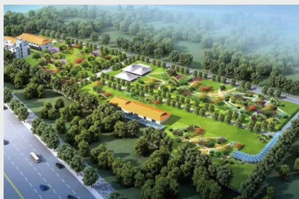
Second Sewage Treatment Plant in Yichuan County, Luoyang City (Treatment Capacity: 20,000 tons/day)
