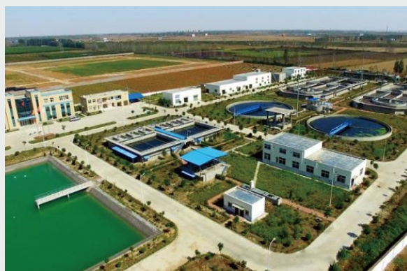
Second Sewage Treatment Plant in Linying County, Luohe City (Treatment Capacity: 30,000 tons/day)
