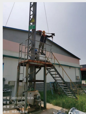
Monitoring of the Hazardous Waste Discharge Outlet
