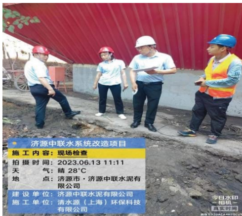
On-site Inspection of the Renovation Project
