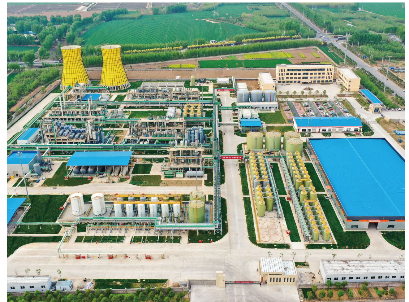
Water Treatment Agent Production Plant of Qingshuiyuan
